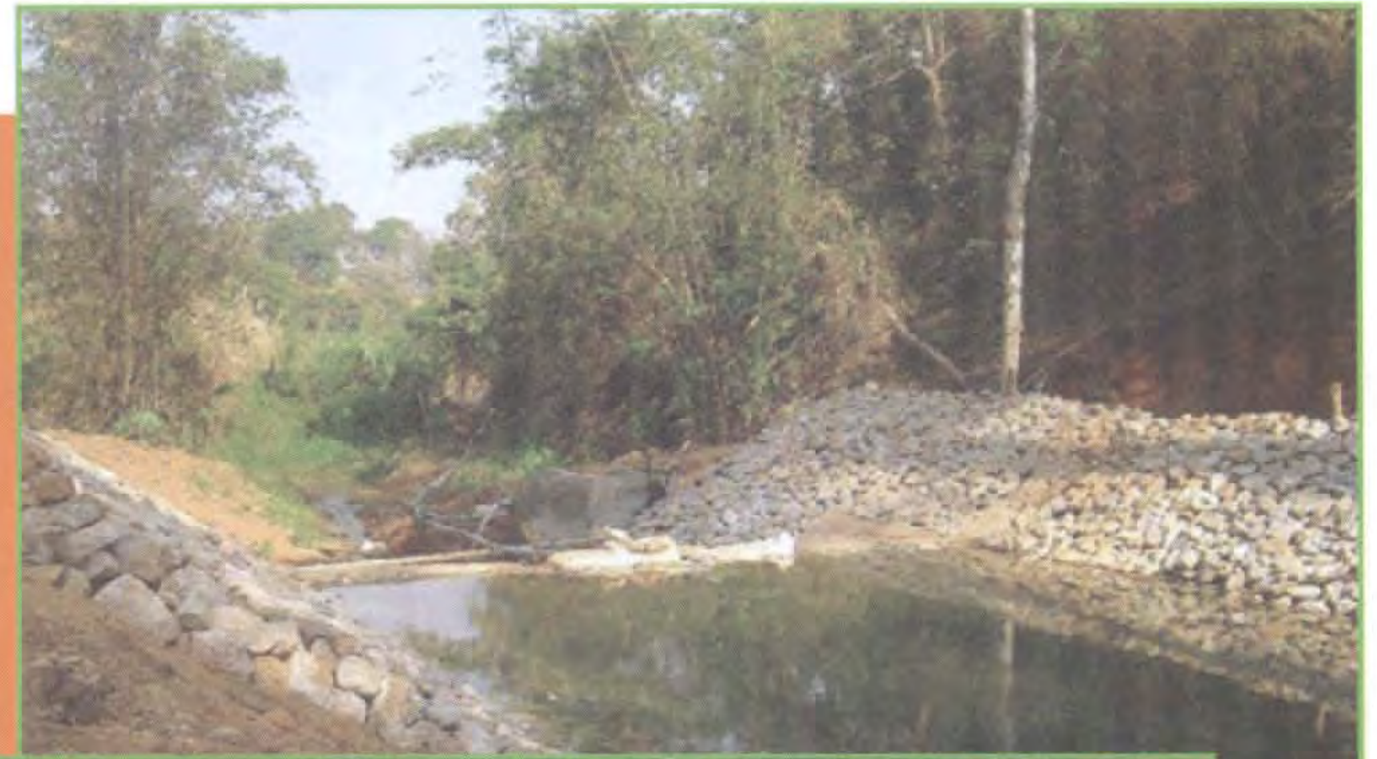
Model pictures of half permanent check dams
