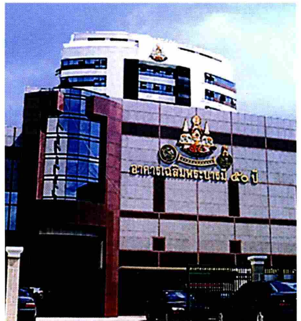
NAGARA BUILDING, BANGKOK
