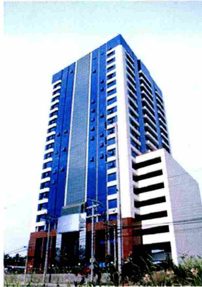
NAGARA BUILDING, BANGKOK
