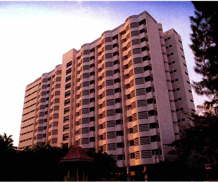
STAFF DORMITORY CHULALONGKORN UNIVERSITY BANGKOK
