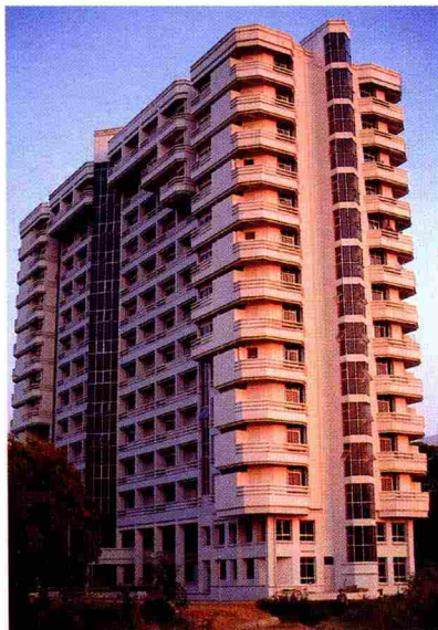
STAFF DORMITORY CHULALONGKORN UNIVERSITY, BANGKOK
