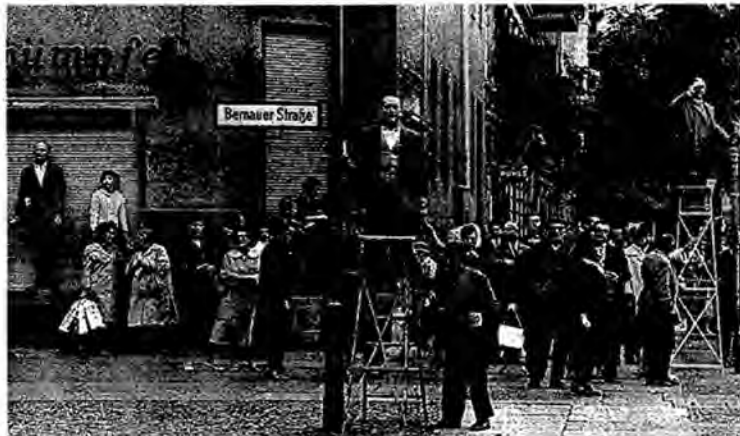
The wall going up on the Bernauer Strasse
