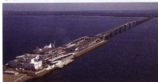
Road Traversing the Tokyo Bay
