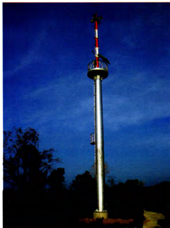
A warning tower
