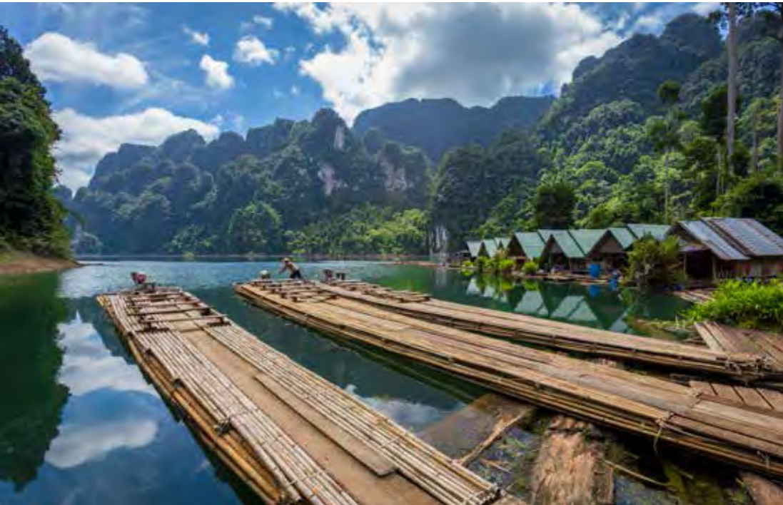
Rajjaprabha Dam or Chiao Lan Dam
